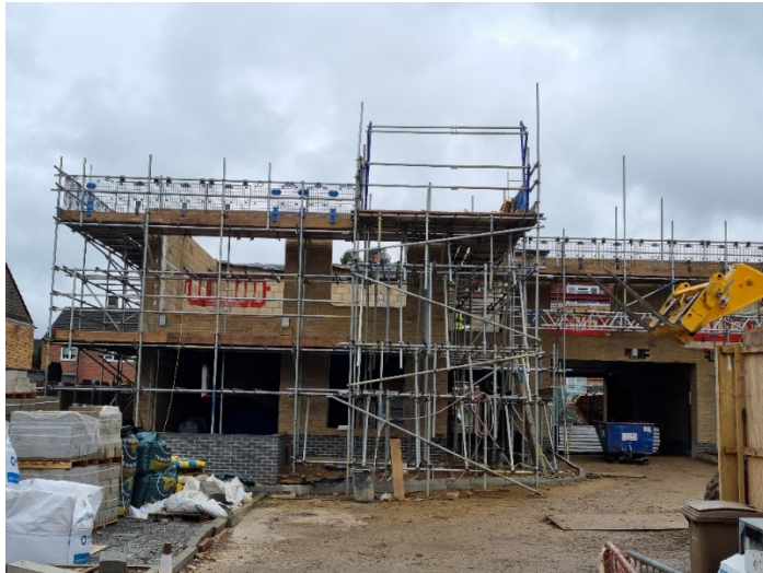
Photo 1 – Construction site at Pentlow Way
