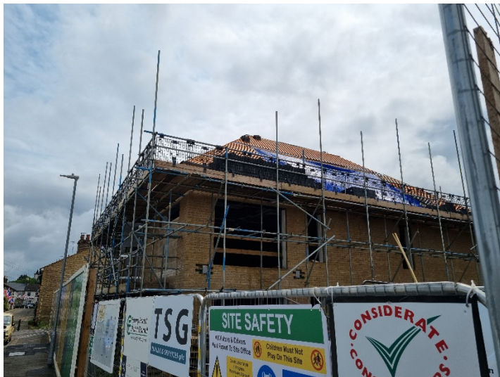
Photo 2 – Construction site at Woollard Street
